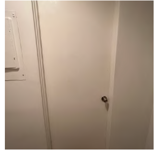
3. SOUTH WALL + DOOR
